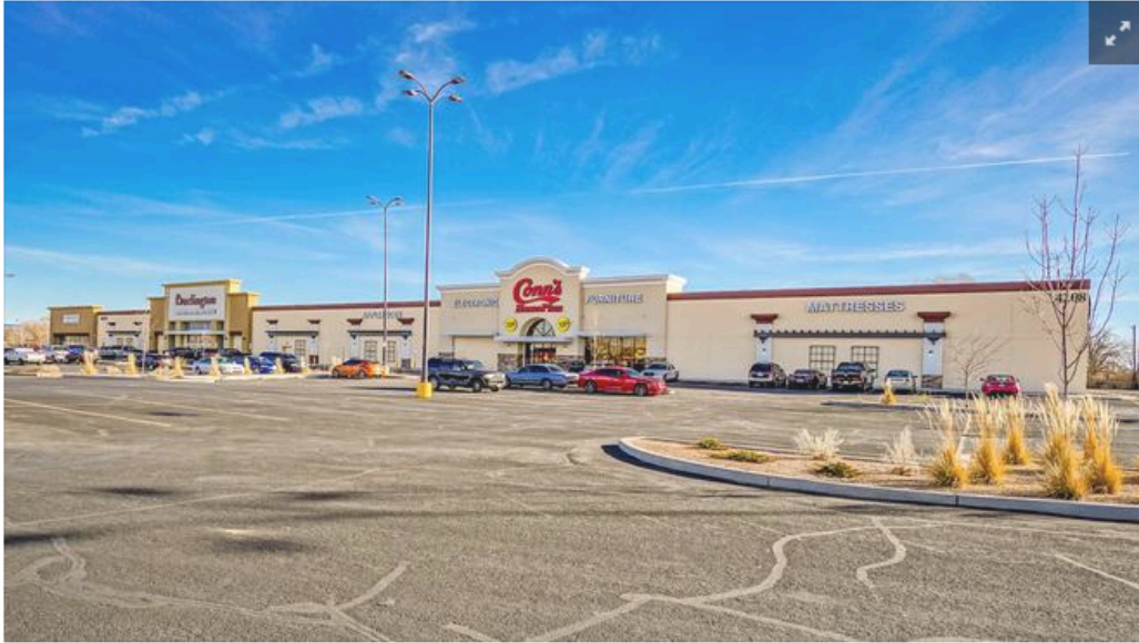
Pictured is the renovated West Central Plaza, located at 4208 Central Ave.
