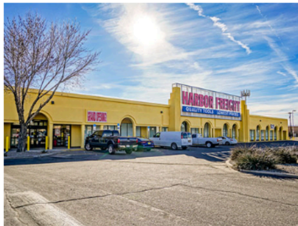
Harbor Freight Tools occupies the converted multi-tenant building at West Central Plaza in Albuquerque.
